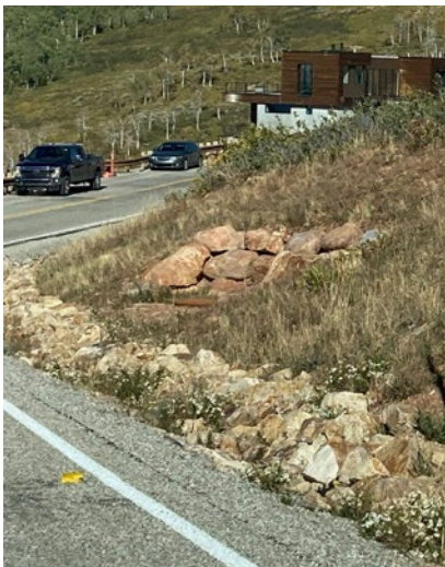
Existing Drainage Swales on Site
